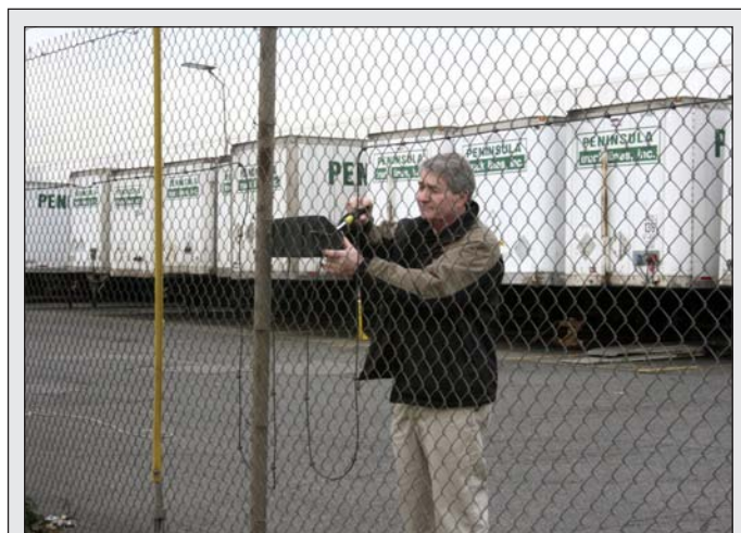
George Nuttle of Security Professionals terminates the INTREPID™ sensor cable at Peninsula Trucking's Portland terminal.
