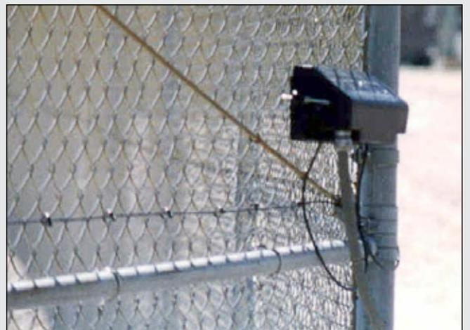
*The MicroPoint Cable perimeter intrusion detection system is preferred by SRP because it works well in Arizona's extreme weather conditions.*
