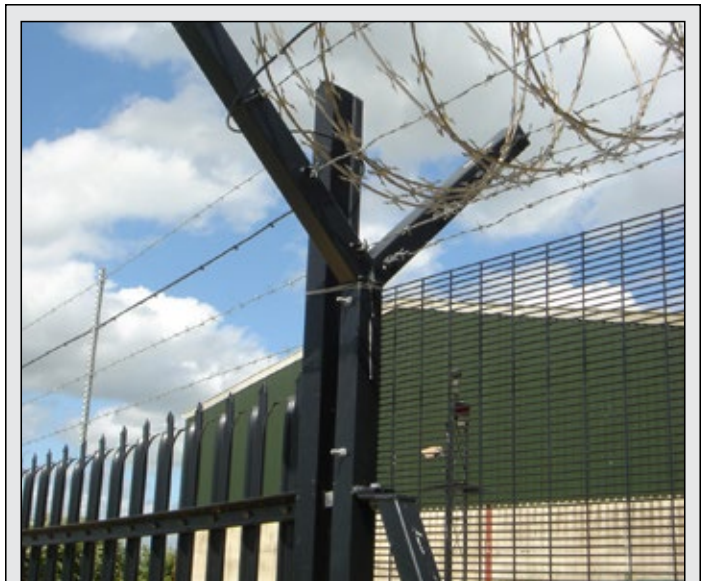
A variety of fence fabric and topping structures are featured to demonstrate a range of European fencing options and the INTREPID™ MicroPoint™ II system’s consistent detection across varying fence conditions.
